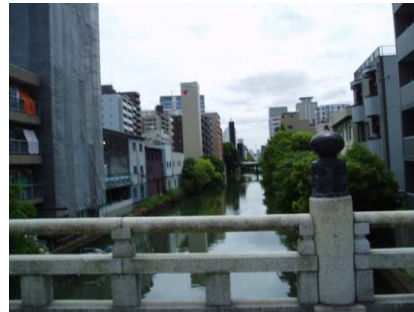
Horikawa River & Gojobashi Bridge
